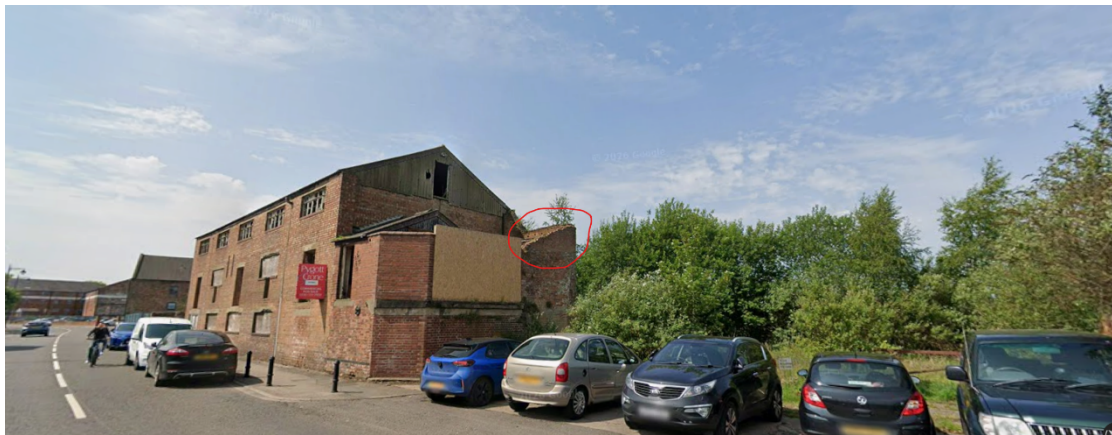
Figure 1 - The immediate relate only to the partial removal of brickwork from the already exposed section of the side structure (as shown in the attached image).
