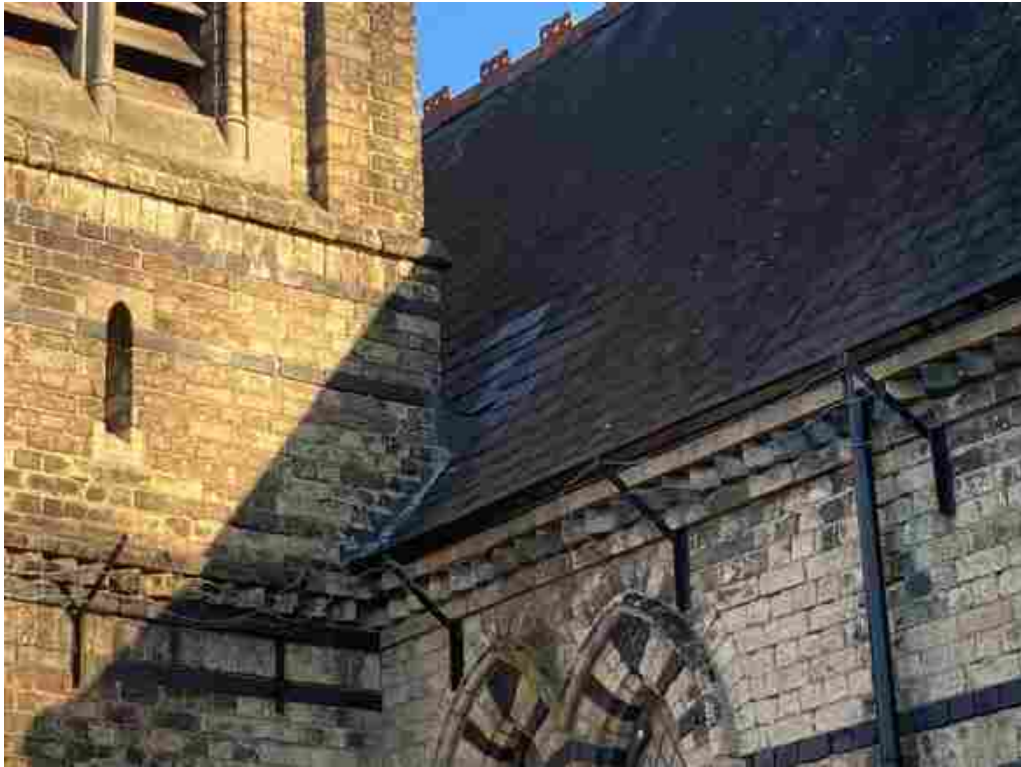
Area of later slates to Tower valley.
