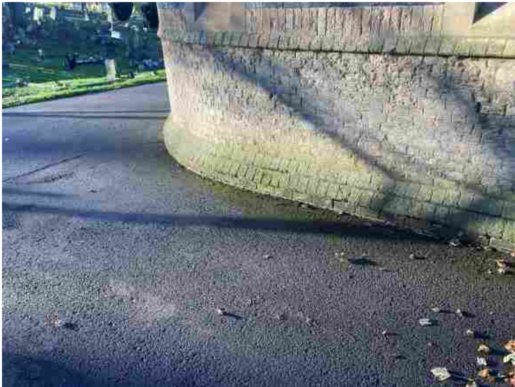
Asphalt has been installed up to the base of the wall, trapping moisture against the building.
