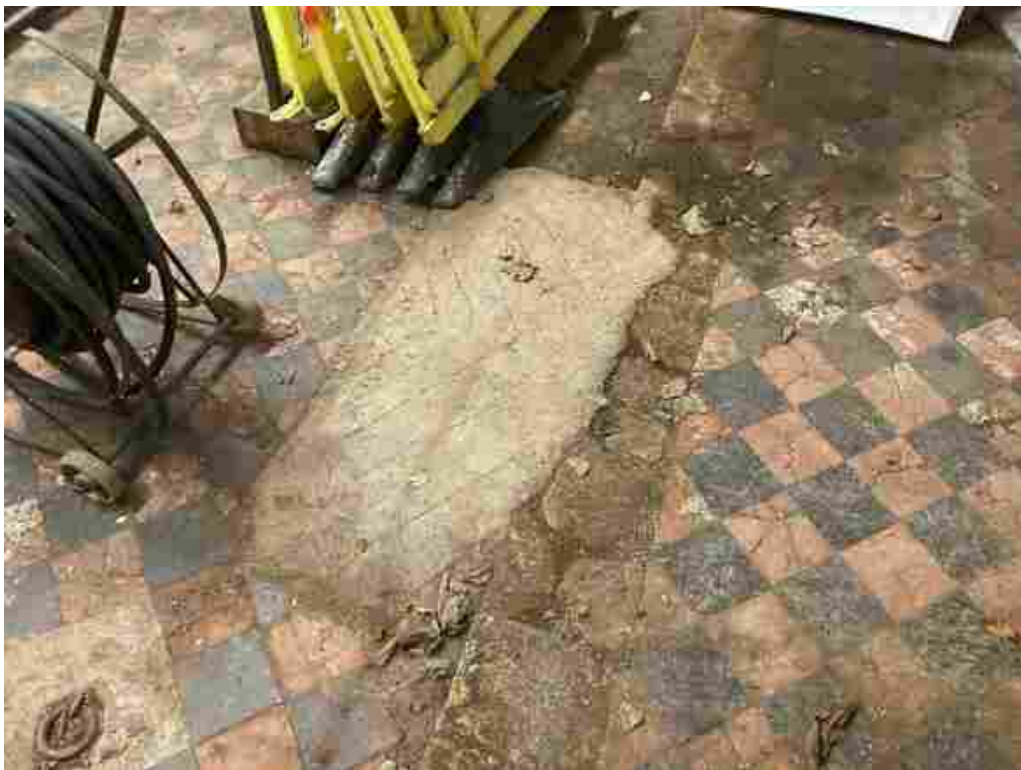
Concrete ramp to overcome change in levels.
