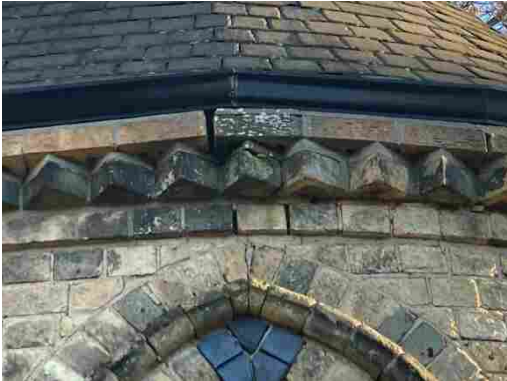
Crack to head of window extending up into the dogtooth brick cornice.
