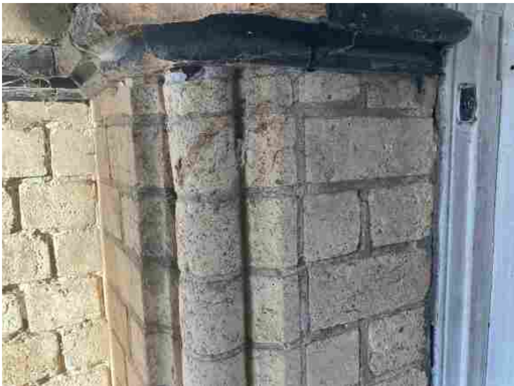
Cementitious mortar to the compound column profile.
