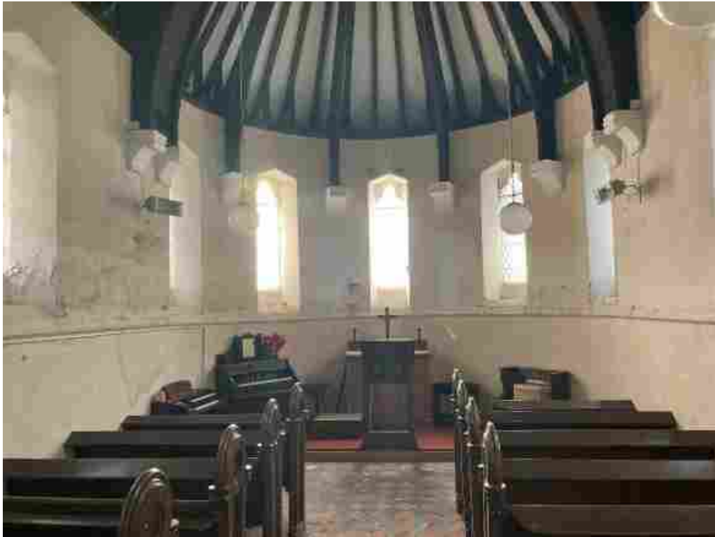
General view of South Chapel interior.
