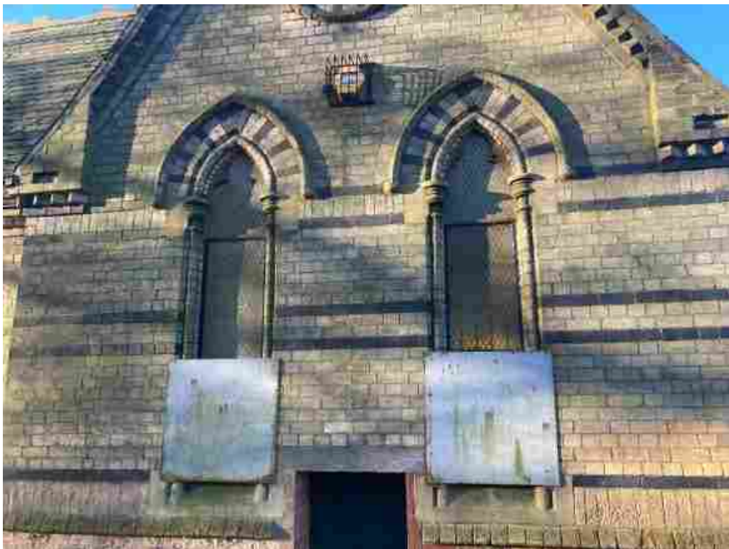
General view of East elevation.
