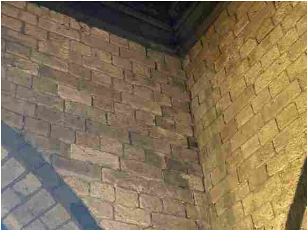
Recessed joints to the Tower base.
