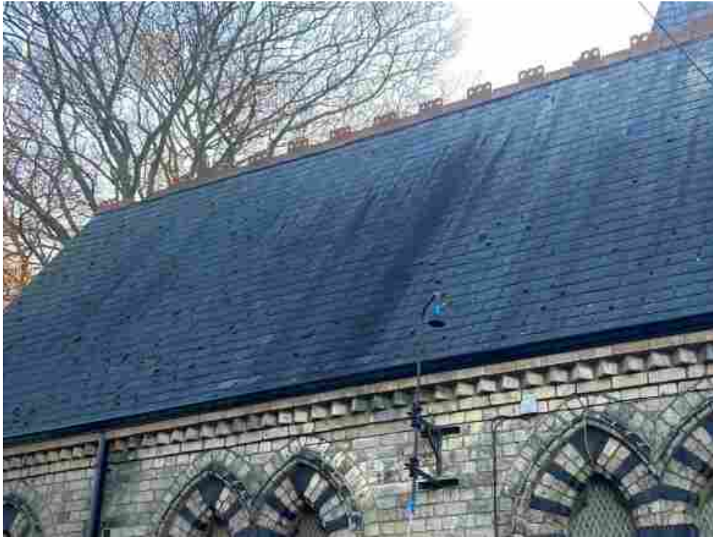
Slating generally appears in satisfactory condition.
