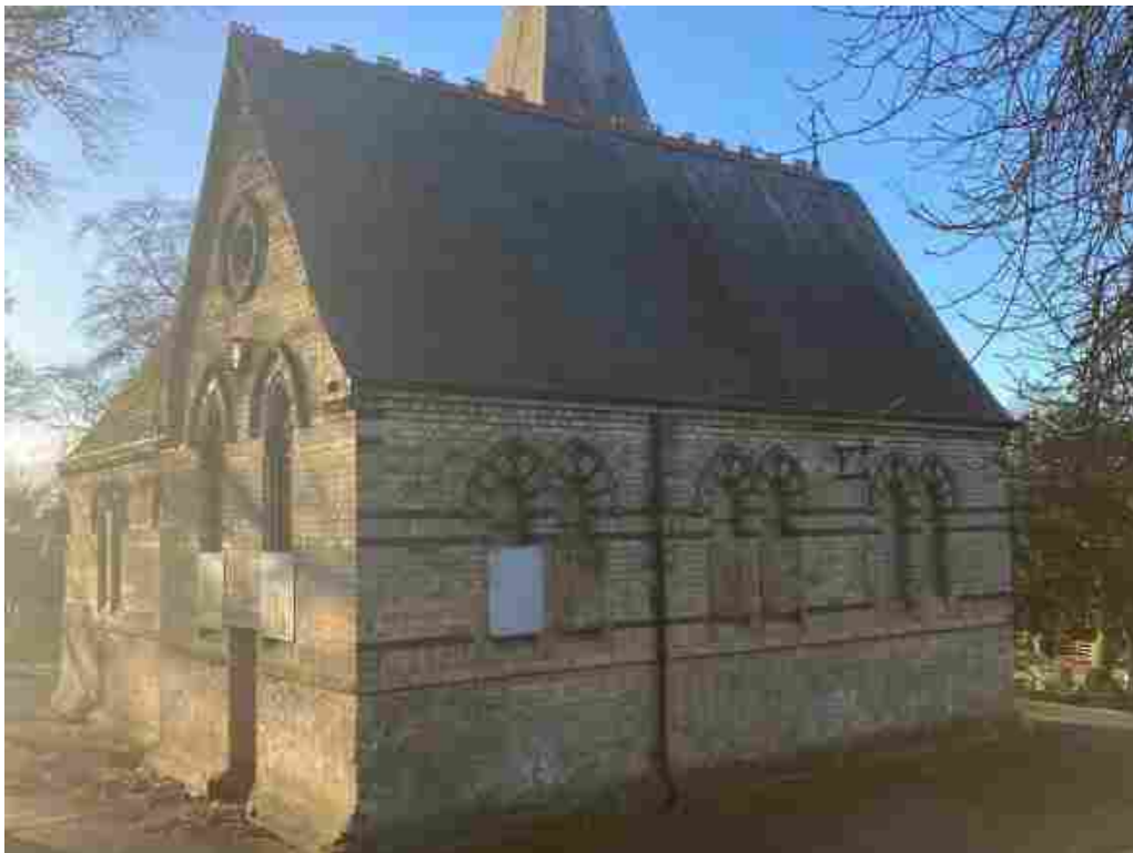
General view of North elevation.
