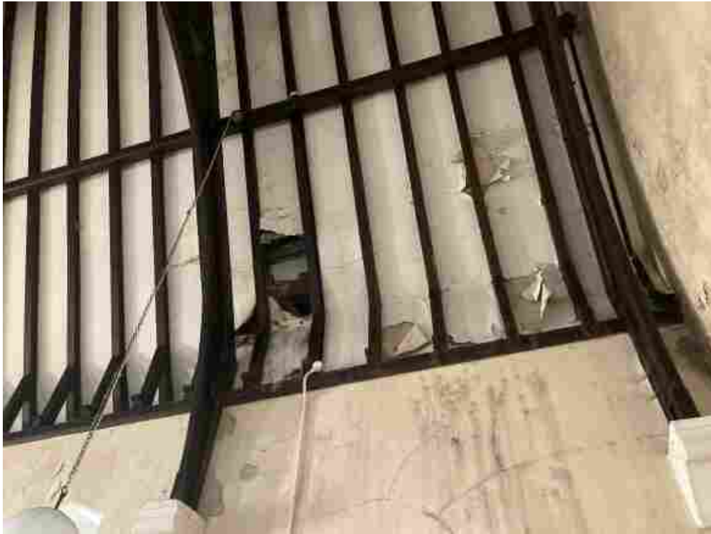
Failing paint and plaster panels to the ceiling.
