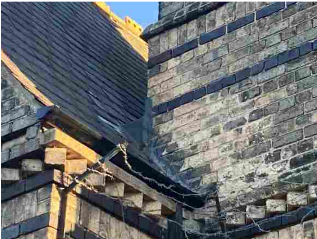
Later repairs to Tower valley.
