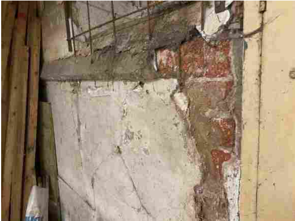
Cementitious render has also been used in this area, which should be removed.
