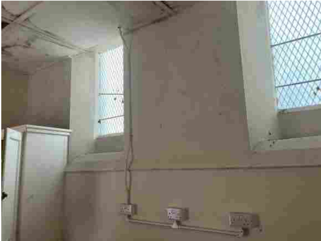
Cementitious render has also been used internally.
