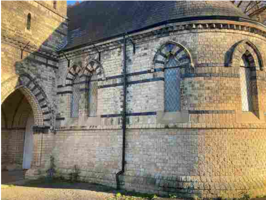
General view of Chapel West elevation.
