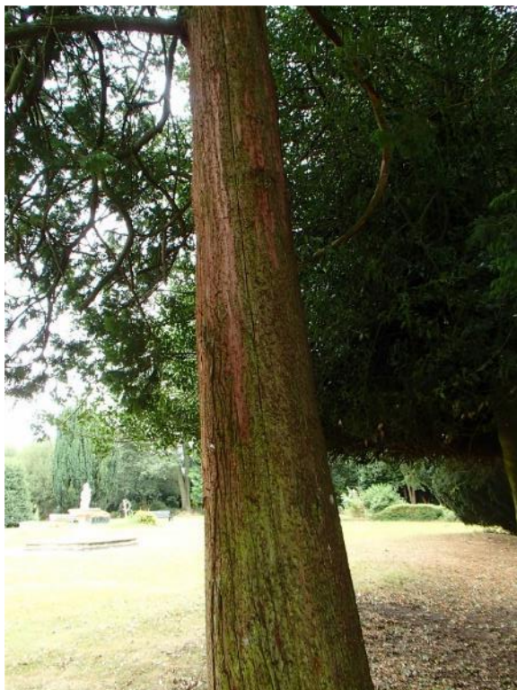
Photo 9: Bark splits on Cypress T79, tree to monitor
