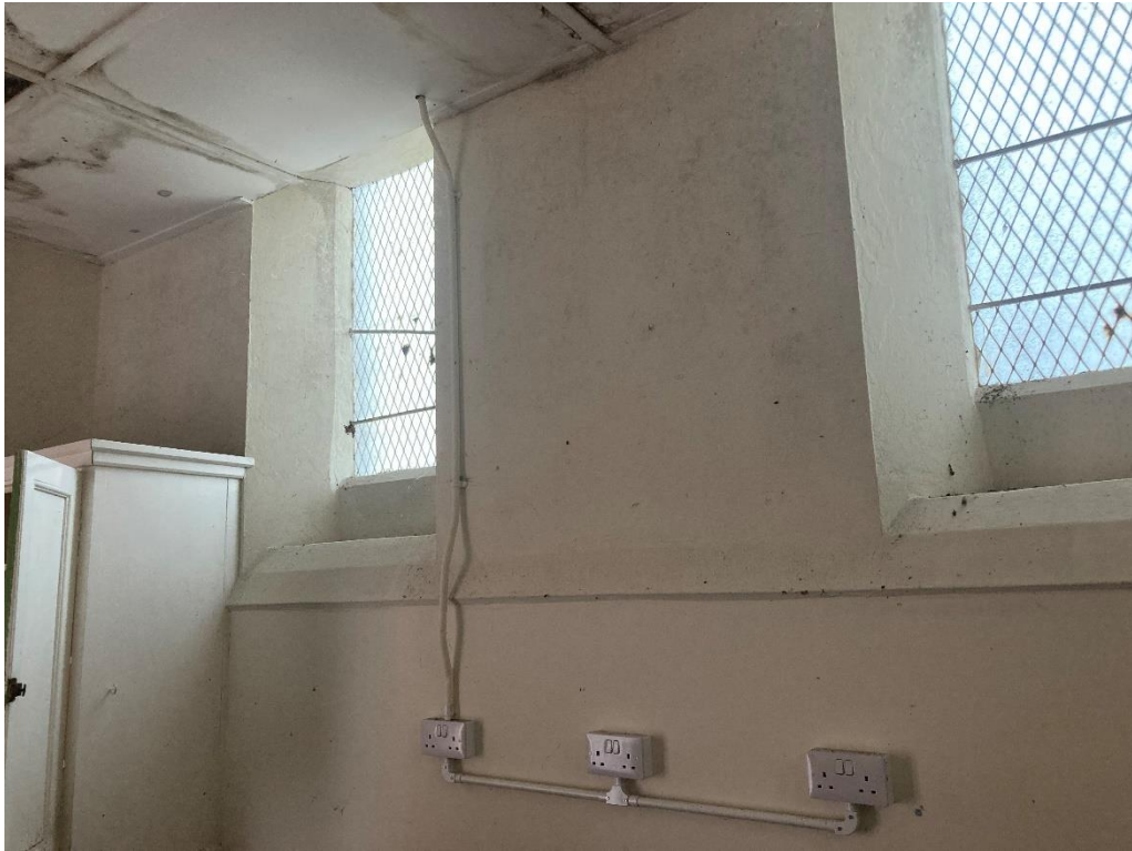
Cementitious render has also been used internally.
