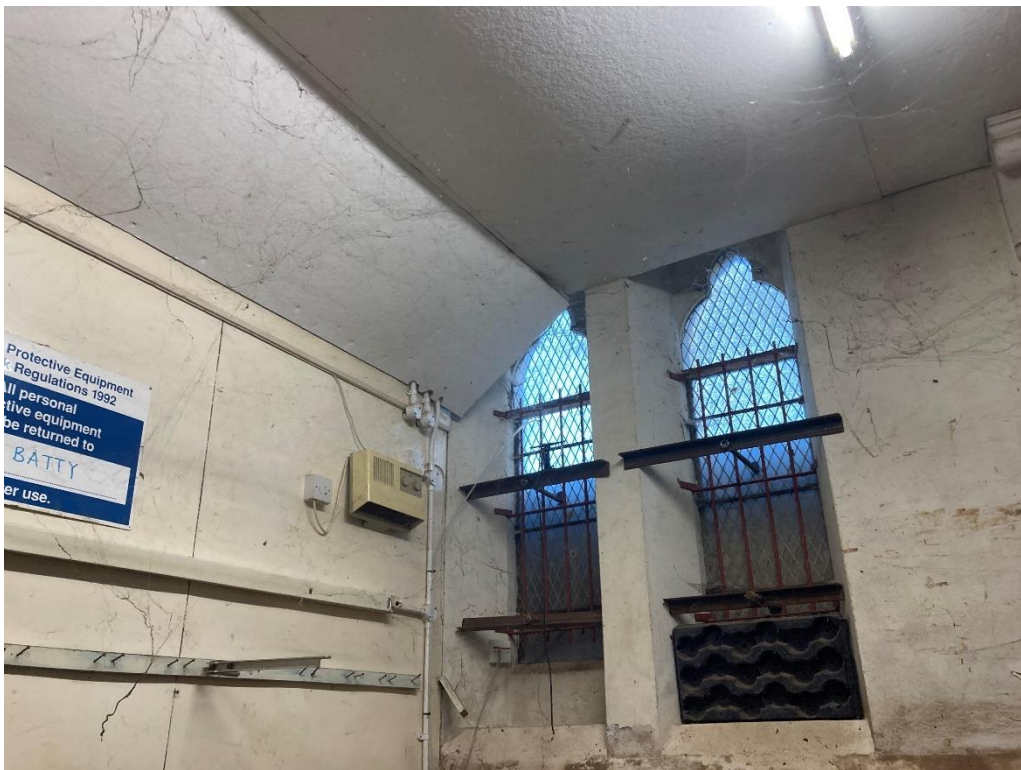
Storage area to North Chapel, subdivided using partitions and ceilings.
