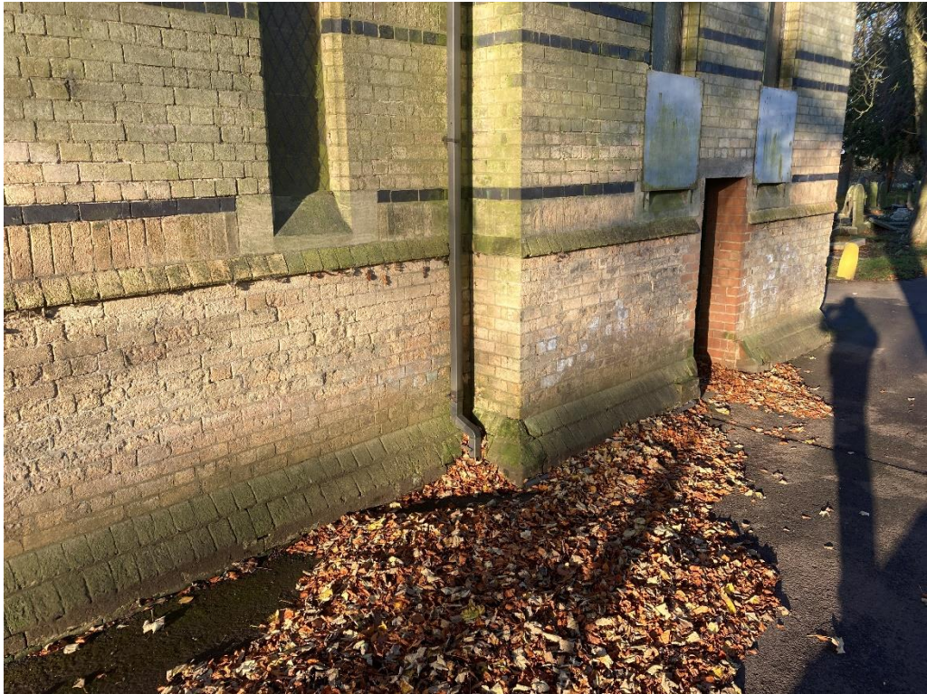
Leaves to gulleys should be cleared regularly.
