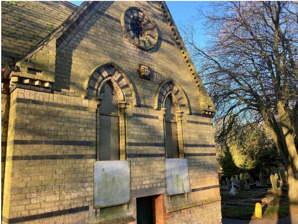
Algaeous growth to East elevation.
