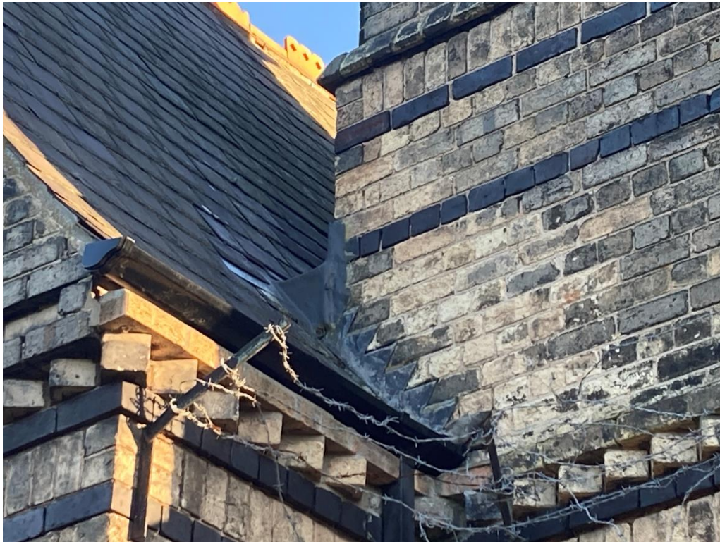
Later repairs to Tower valley.
