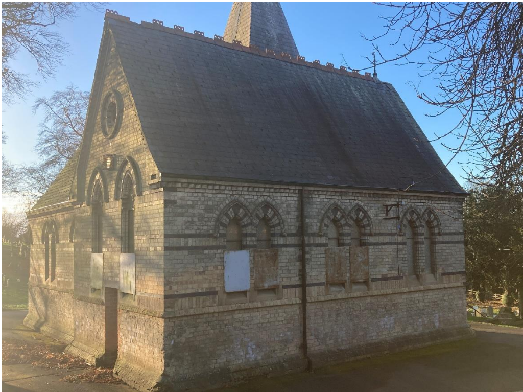
General view of North elevation.
