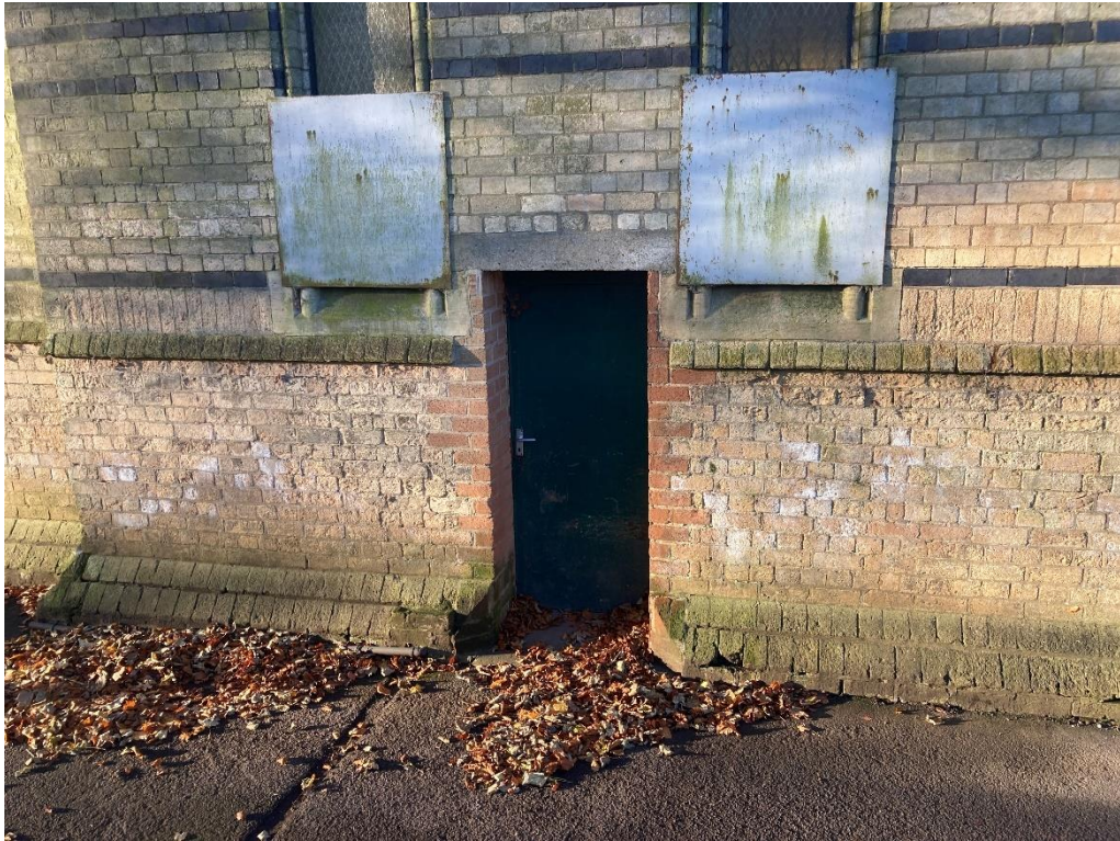
Later alteration of East elevation to introduce door.
