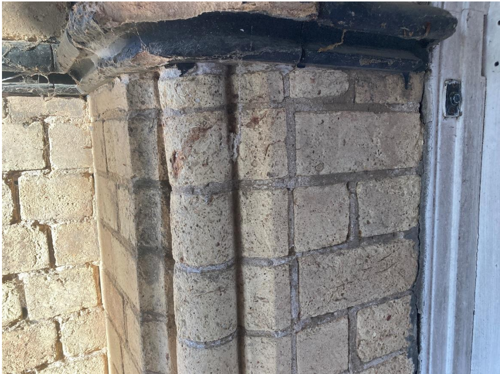
Cementitious mortar to the compound column profile.
