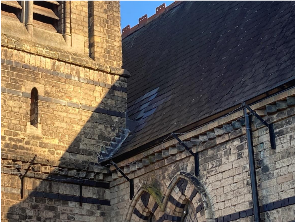
Area of later slates to Tower valley.
