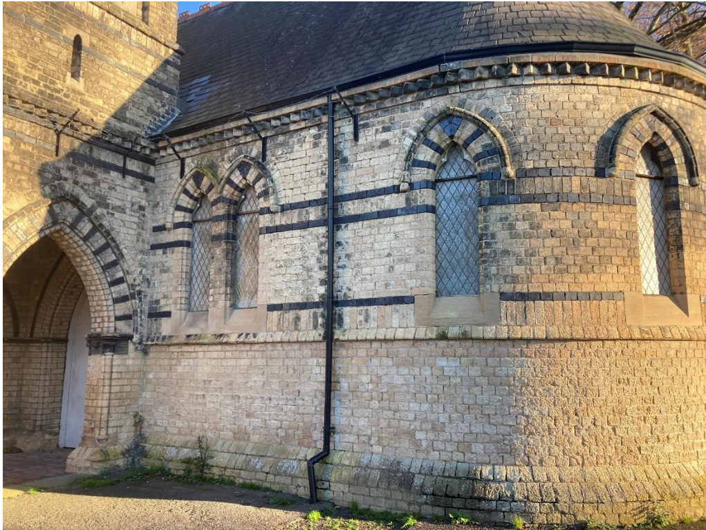
General view of Chapel West elevation.
