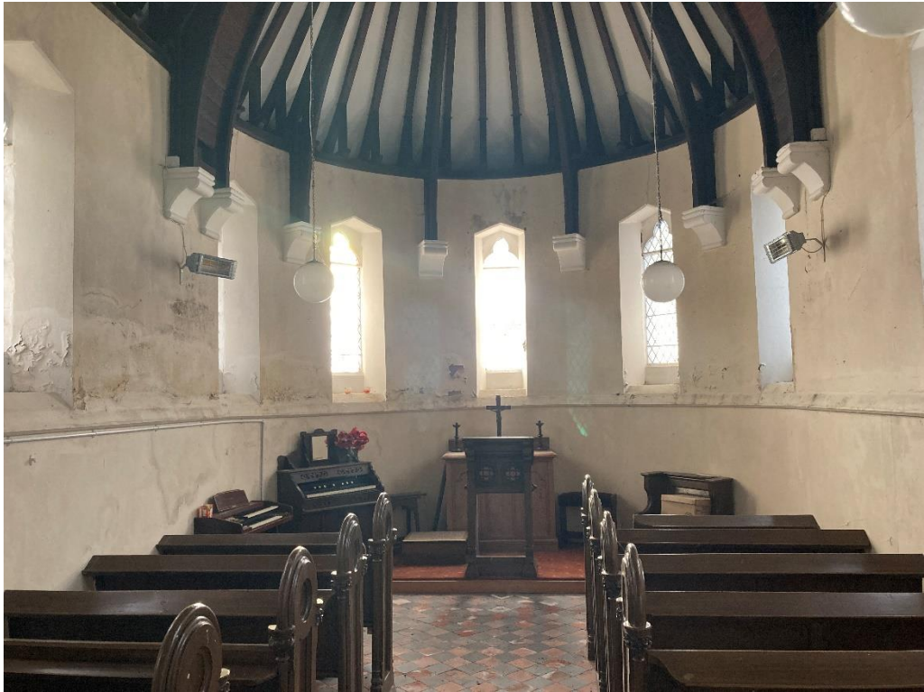
General view of South Chapel interior.
