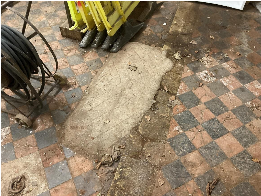
Concrete ramp to overcome change in levels.
