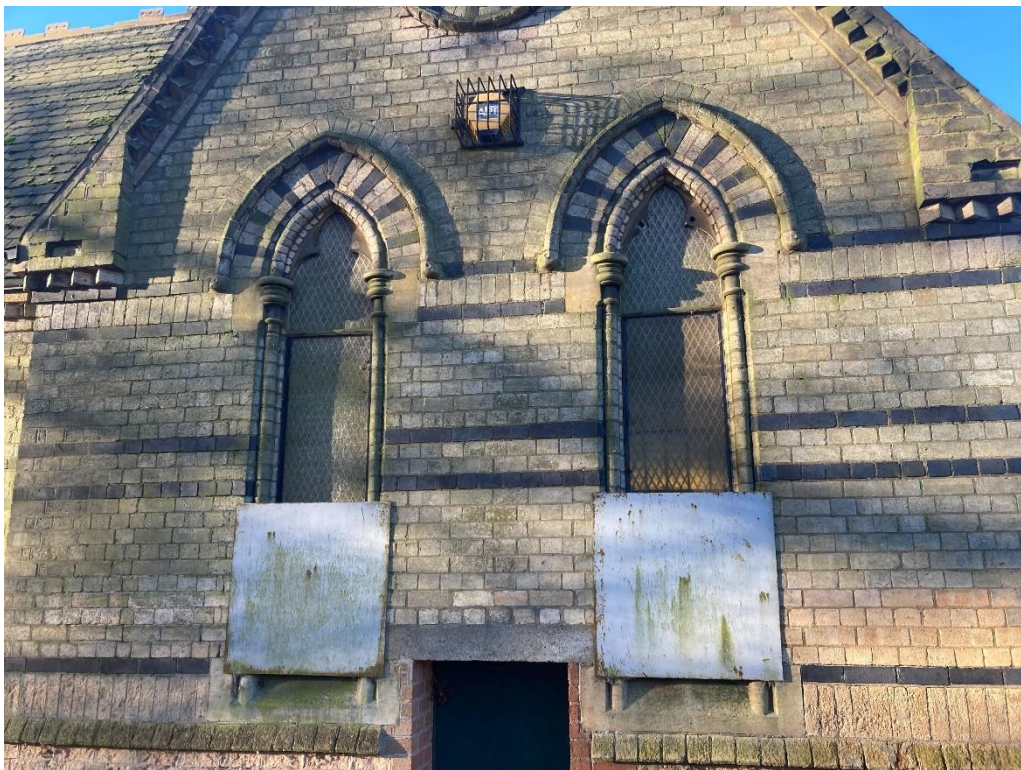
General view of East elevation.
