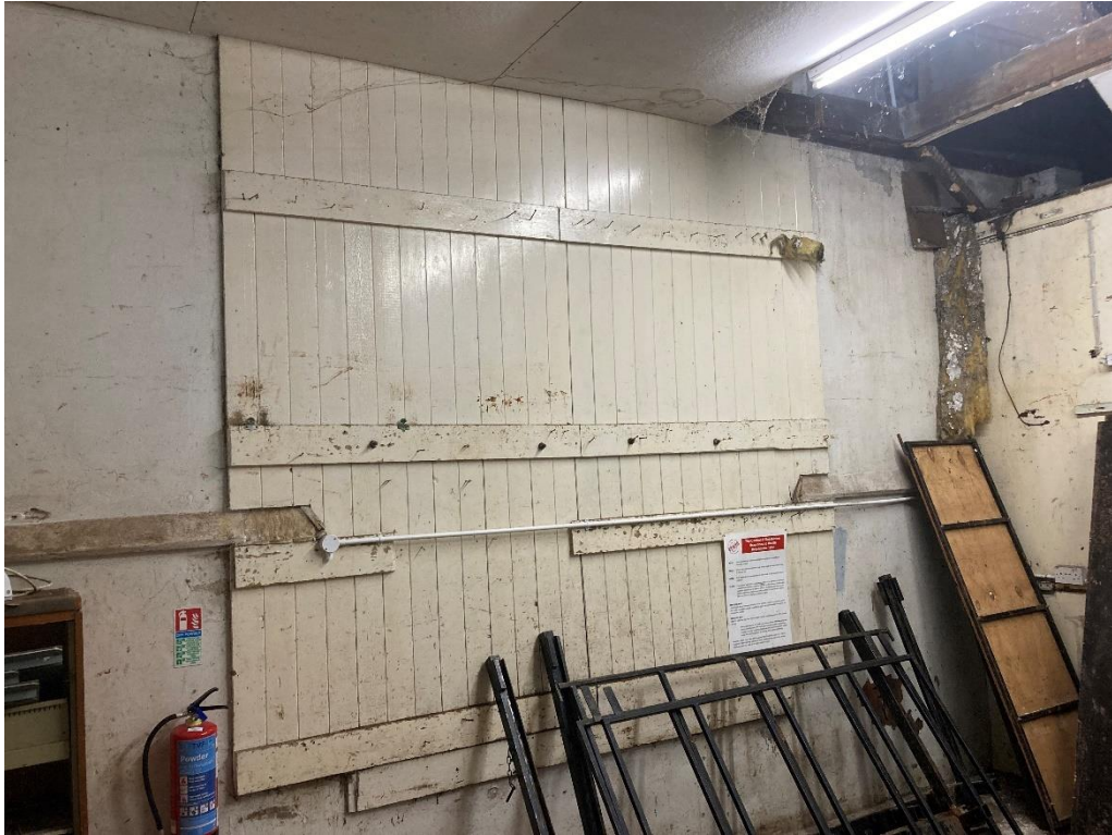
Timber boarding between the North and South Chapels.
