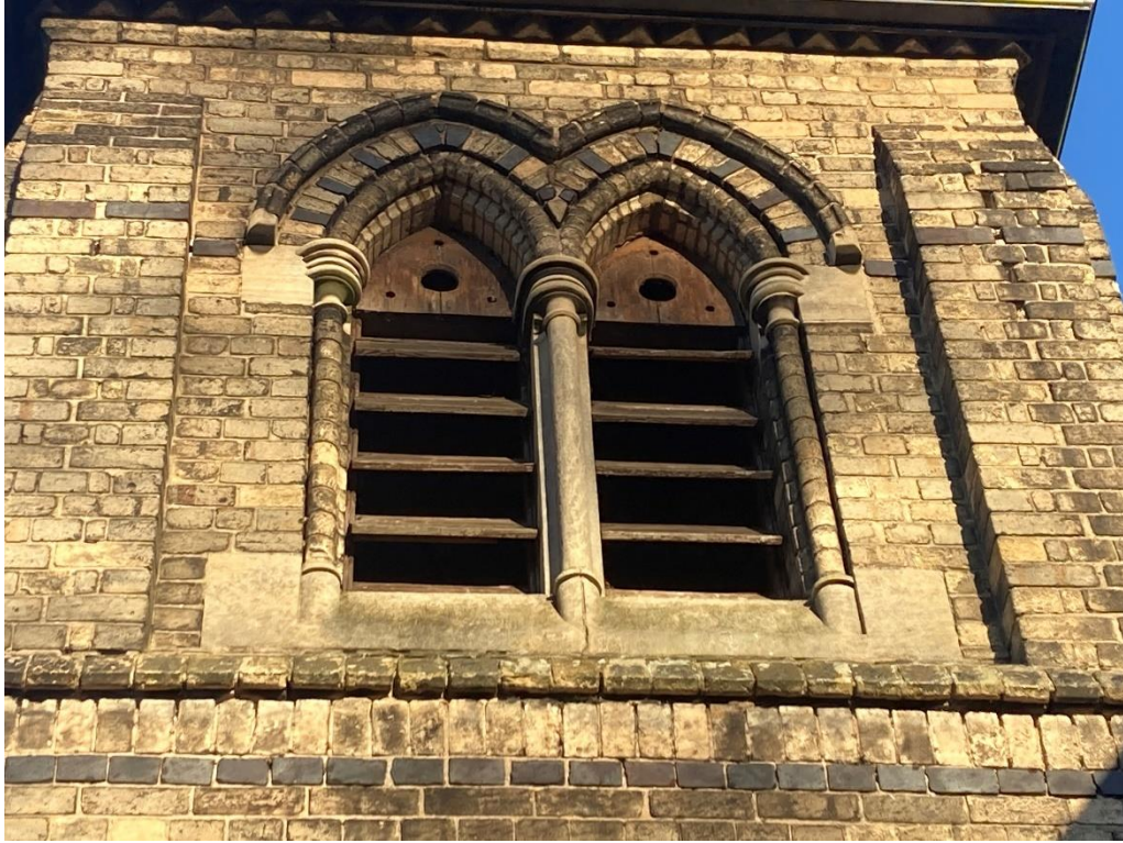
Belfry louvres could be meshed, repaired and redecorated.
