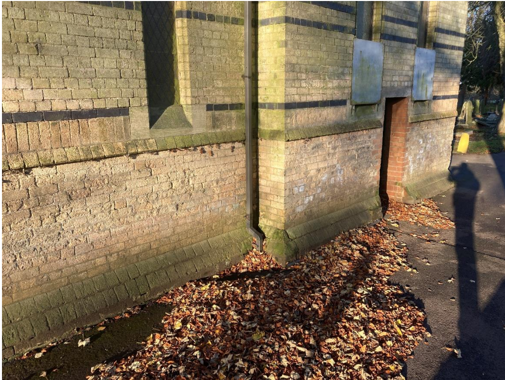
Leaves to gulleys should be cleared regularly.
