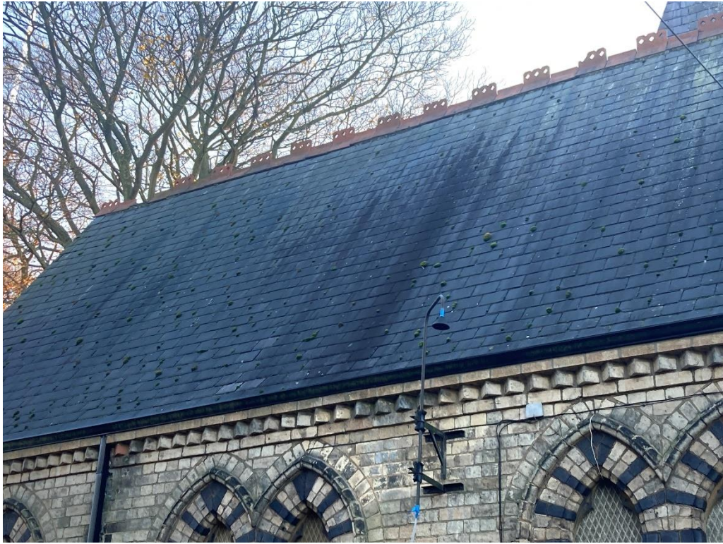
Slating generally appears in satisfactory condition.
