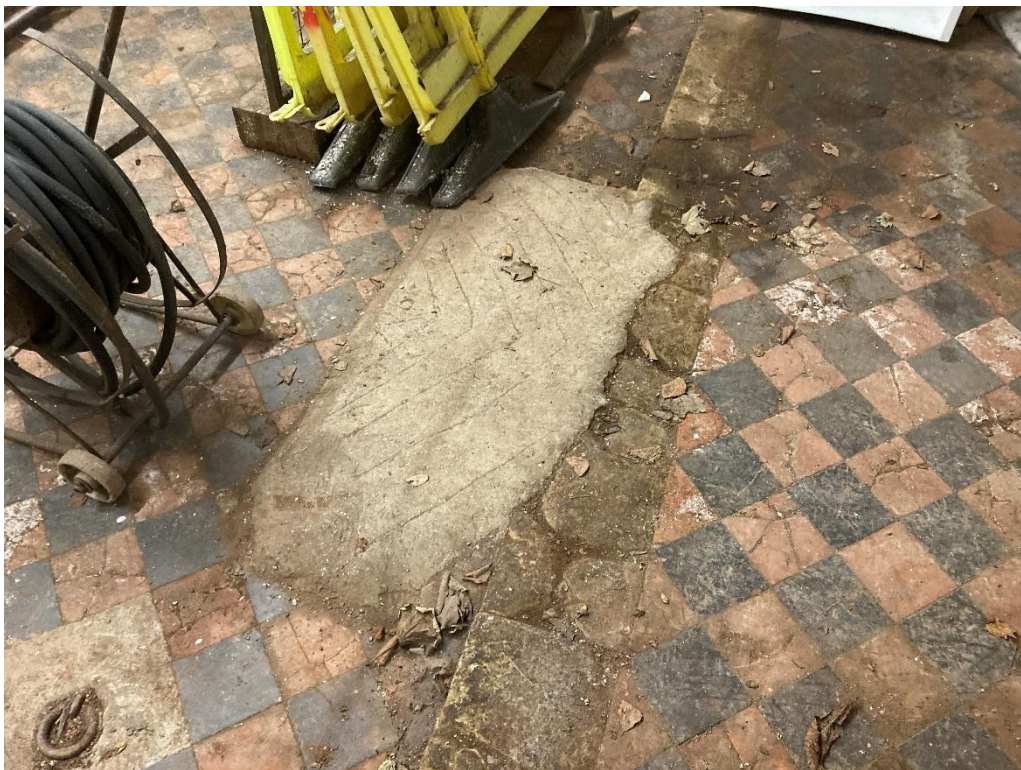
Concrete ramp to overcome change in levels.
