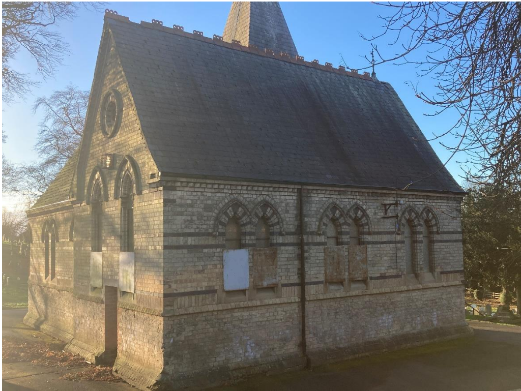
General view of North elevation.
